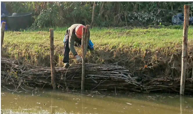
Figg. 21, 22. Posa delle fascine / Laying the fascines
