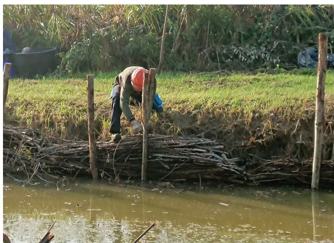
Fig. 21, 22. Posa delle fascine / Laying the fascines
