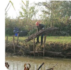
Over 300 meters of internal channels have been dredged to improve the exchange of water with the large ponds of the Oasis; 9 sluices were replaced to improve water circulation; installed sensors to control water levels; install fascines to protect 500 meters of banks from erosive phenomena. Water control favors the project's priority habitats and regulated flooding will control the presence of *Rubus* spp. and *Robinia pseudoacacia*.
